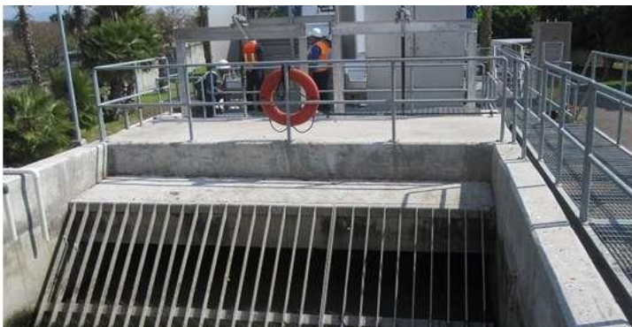
Figure: Coarse Screen
