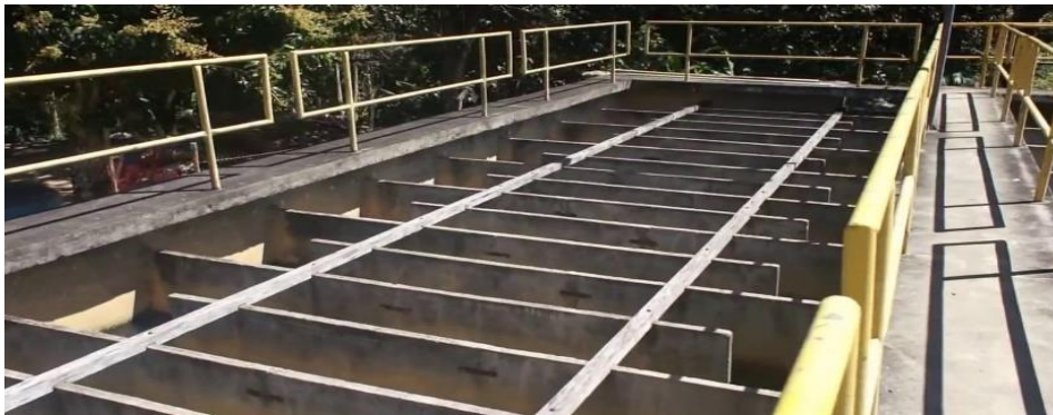
Figure: Horizontally Baffled Tank Flocculation
