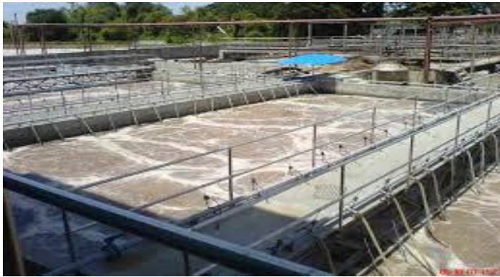
Figure: Aeration Process
